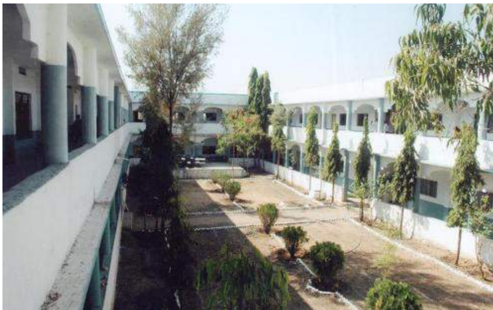
Maintenance work for greener campus during lockdown (Covid-19)
