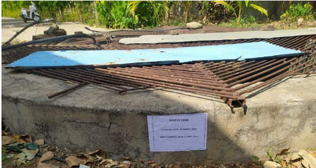
Underground water tank
