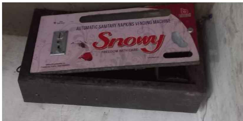
Installation of Sanitary pad vending machine for girls
